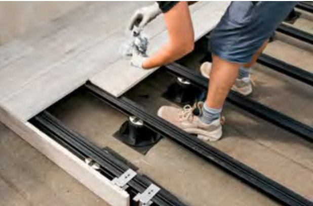
STEP 4 Use the spacers from the kit, in order to lay down the tiles properly.
