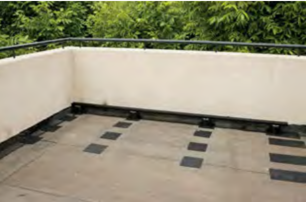
STEP 1 Put the mute mats and the supports into position on the floor (perimeter support must be cut).
