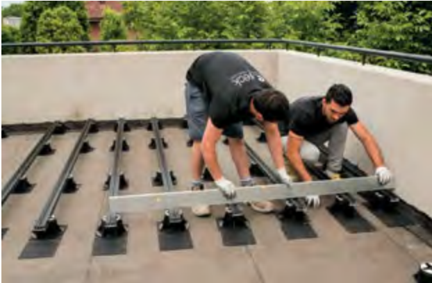
STEP 2 Put the joists into position (12" in-between) and secure them by pressing them down gently.
