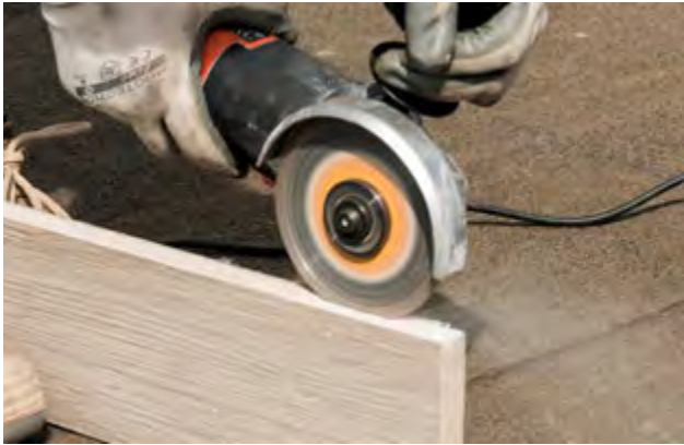
STEP 6 Cut on the edge of the slabs, in order to fit them into the lateral restraint.
