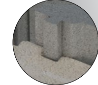
Tenon and mortise on one side
