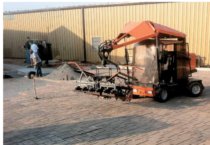
Paver laying machine
