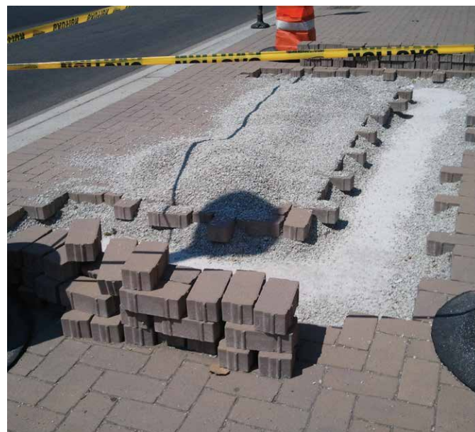
Pavers being removed to allow for an underground repair.
