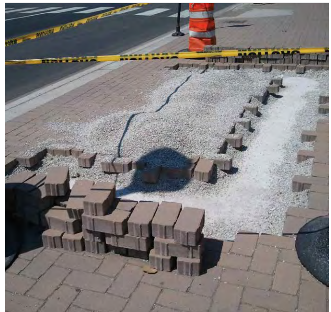
Pavers being removed to allow for an underground repair.
