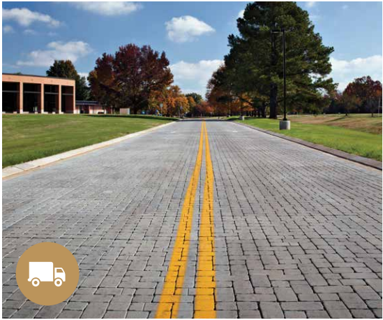
Occasional Heavy Vehicles Designated for vehicular areas, parking lots, and roadways where limited heavy vehicles are anticipated daily such as large delivery trucks or garbage trucks.
