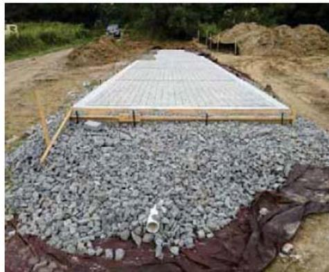
Figure 2-2: Test pad following construction (Aug 18<sup>th</sup>, 2017).
