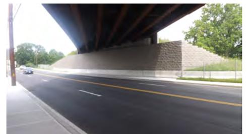
Geosynthetic Reinforced Soil (GRS) consists of free-draining, high-quality granular backfill combined with closely spaced layers of medium to high strength geogrids or geotextiles. The main factor that makes these types of construction so attractive to states, counties, and municipalities is the reduction in construction time and overall costs. These types of bridges are used as road overpasses and over waterways with spans up to 140 feet.
