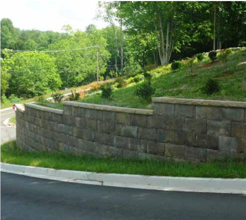
This road-widening project butted directly up against the homeowner's yard. Mega-Tandem™ MSRW™ System provided the structural integrity needed for the city, as well as pleasing aesthetics for the resident. Mega-Tandem™ MSRW™ System also eliminated the need for a geo grid and saved the city from having to seize more of the homeowner's property through eminent domain.
