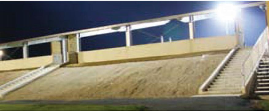
The seating system was constructed from the ground up, starting with a compacted base fill that was graded to the correct pitch.
