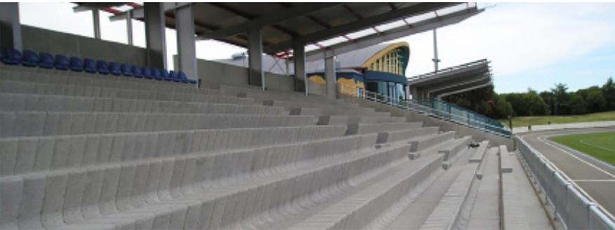
After a concrete slab was poured on the graded bases, concrete seating modules were installed, consisting of separate Seat blocks and Step-Aisle blocks. Individual blue plastic seats were bolted to the concrete Seat blocks, allowing for easy seat replacement if damaged from use.
