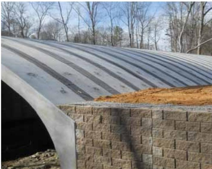
**Bridges were constructed with massive, 50-foot-wide arch culverts and the Vertica Stone Cut retaining wall system.**
