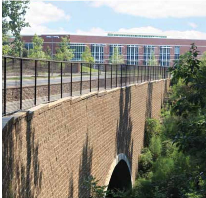
**The Vertica Stone Cut<sup>®</sup> retaining wall system integrates with arch culverts to preserve wetlands and support three road bridges.**
